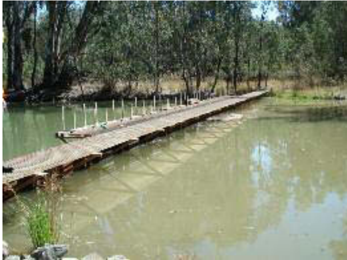
The fourth Moira Lake regulator installed by the Working Group
