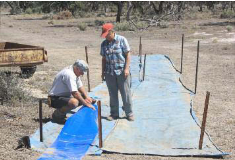
Ken and Anne Warren set up the new lay-flat piping in preparation for pumping water into wetlands at Wingillie Station
